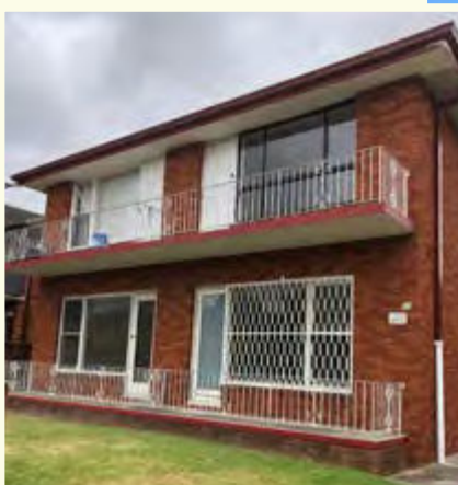
Campsie Block before Refurbishments
