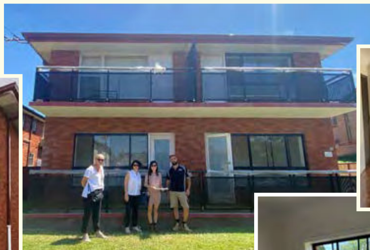
Campsie Block during Refurbishments
